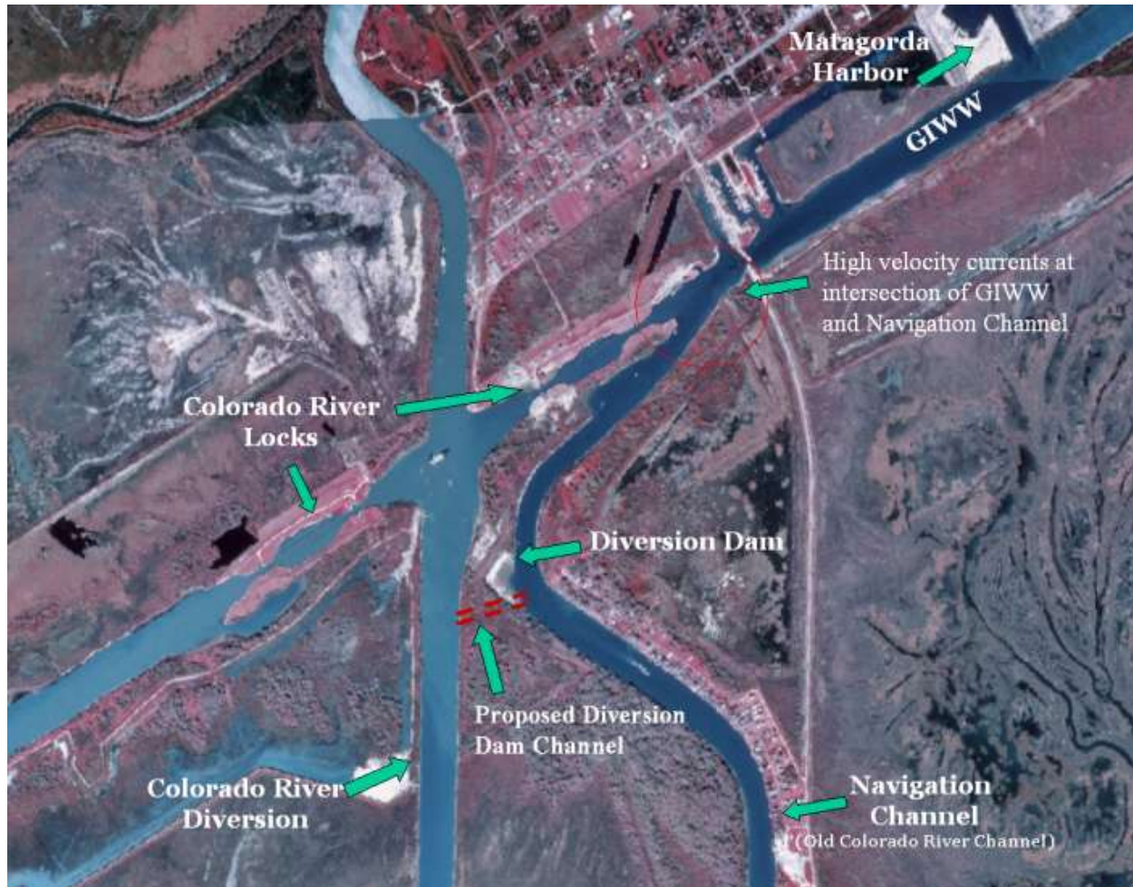
Figure 2.14: Colorado River Diversion Channel and Navigation Channel
